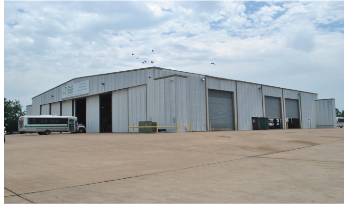
Brazos Transit District building, Bryan, TX.
